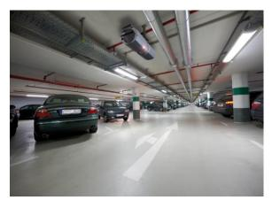
Most countries have developed a national standard for car park ventilation or have adopted legislation to cover the minimum requirements. Most countries distinguish two functions for the ventilation systems. A base function is air refreshment to comply with the max. permissible pollution limits. A second function is usually the extraction of smoke and heat in the case of fire. In order to achieve a trouble-free system and maximum operating safety, all system components have to match perfectly.
